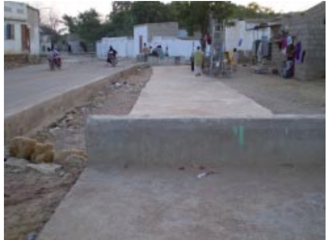
Sewers run beneath this concrete pathway
